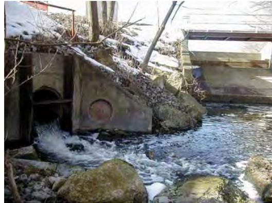
*Photo 4-3: LaPorte main WWTP Outfall 001 on left and CSO Storage Lagoon Overflow Outfall 002 on right*
